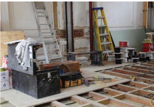
Cable installation in progress
